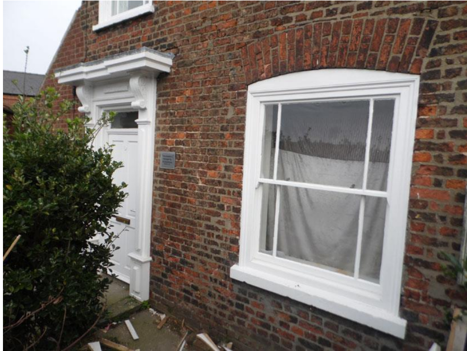
The existing ground floor window with its segmental arch and cill on No.2 Skirbeck Road; typical of all of the street façade windows on the building.
