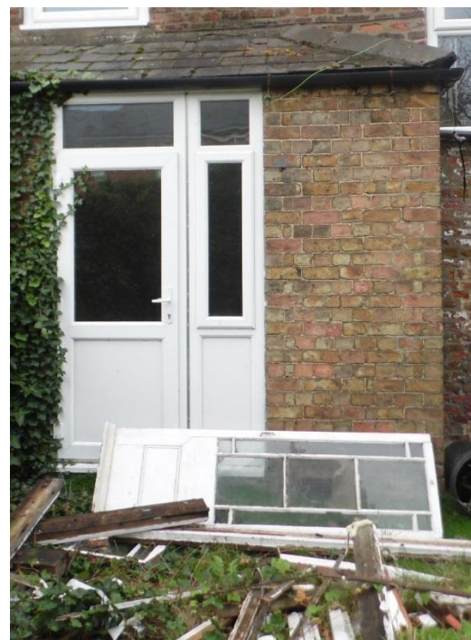
The existing historic rear ground floor double doors recently removed but still on site. To be reinstated.
